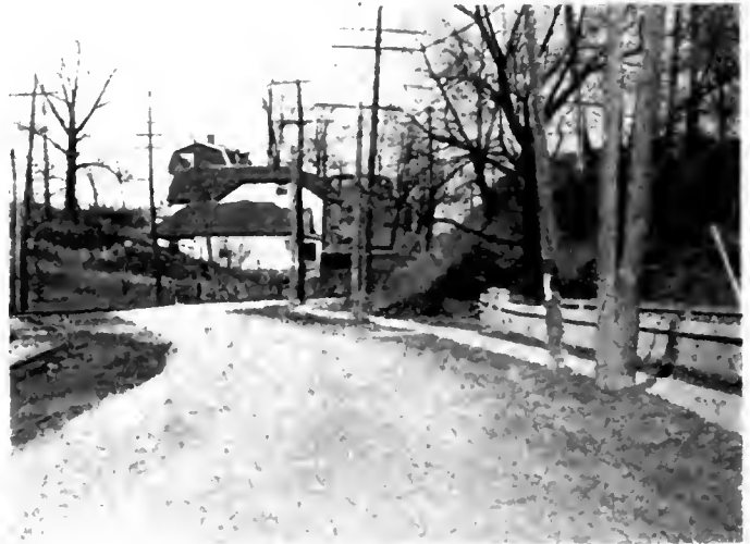
Fig. 4—A reverse curve and a high bank made this a dangerous spot.
